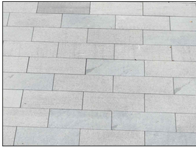
CODE: PV02 DESCRIPTION: UNIT PAVING FINISH: 600x300x40mm STONE GRANITE
