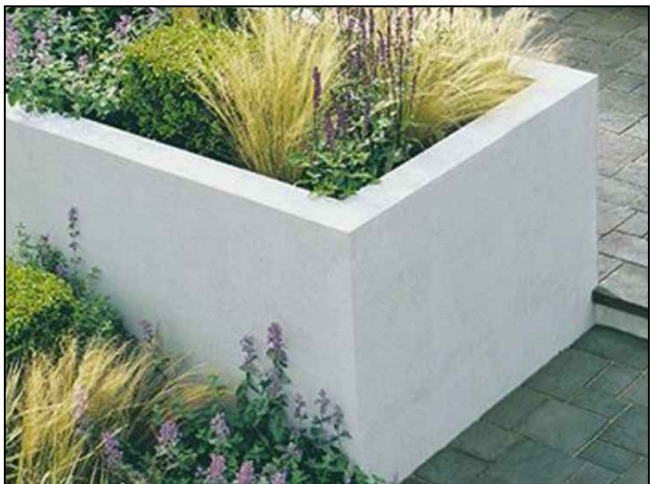
CODE: WA02 DESCRIPTION: MASONRY CORE FILLED BLOCKWORK WALL FINISH: RENDERED FINISHES
